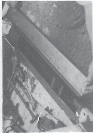
FIG 3 Door tread plate replacement - rivetted panel
