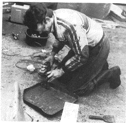
Dressing the replacement floor prior to refitting.
