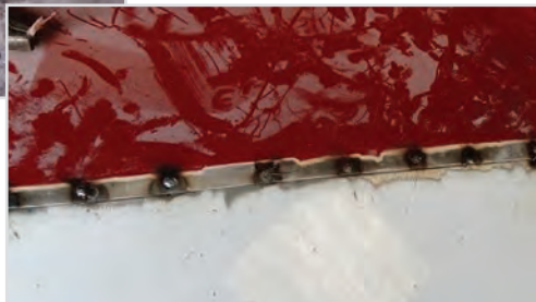
Plug Welds for Minimal Distortion
