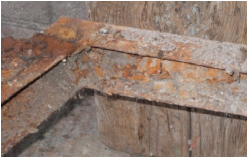
Typical rusty area of the outer side rails.
