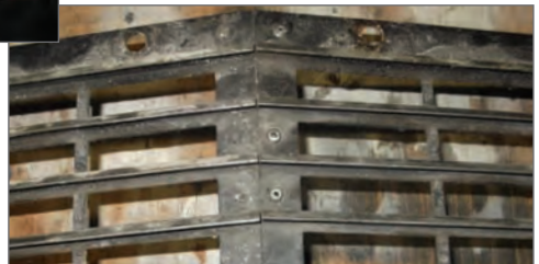
Front Grill re-riveted
